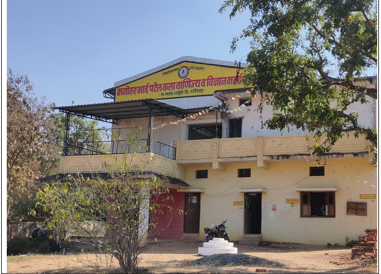
COLLEGE BUILDING FRONT VIEW
